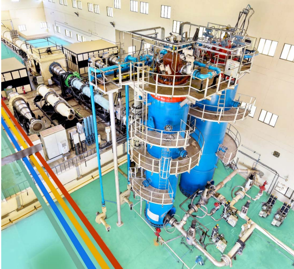
Photograph of 1m Hypersonic wind tunnel facility
